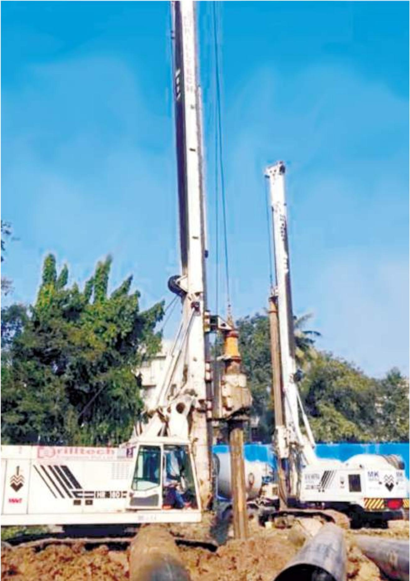
Permanent M.S. Liner for 700 mm Diameter of pile at **PATEL REALTY**
