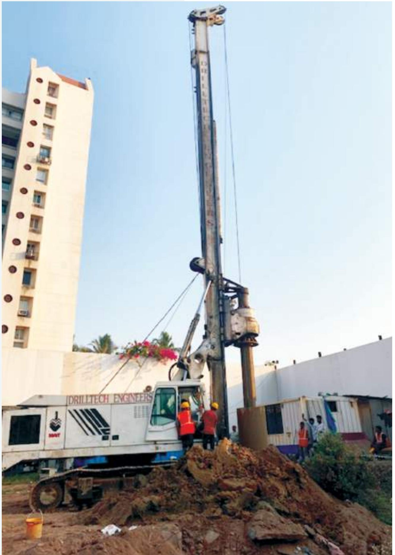
Permanent M.S. liner for 900 mm diameter pile 29 mtr. Depth at Darya Mahal Versova, **RADIUS DEVELOPER**
