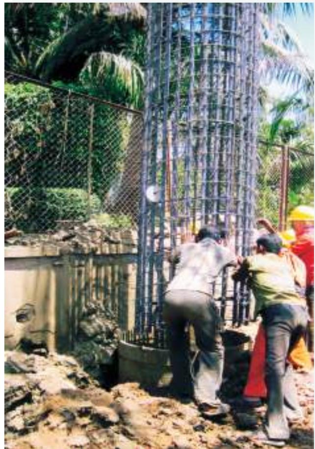
Cage Lifting by Crane & Lowering into the 1500 mm Dia Piles
