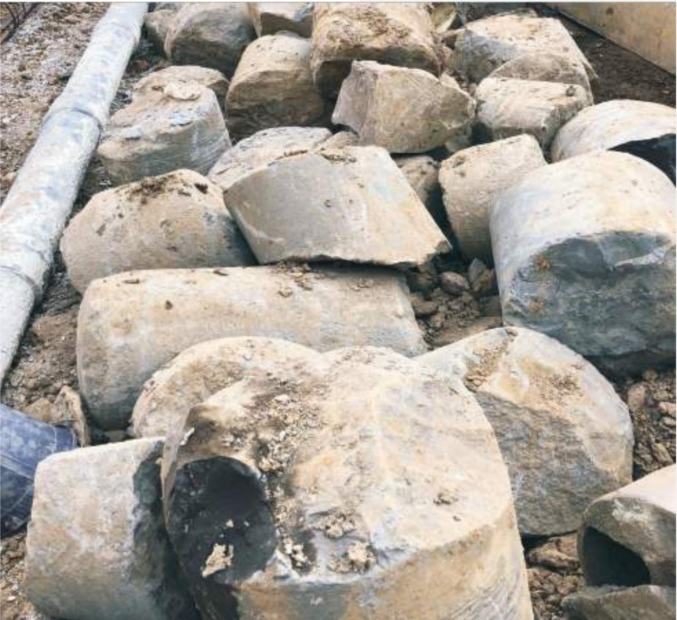
Basalt Cutting with Core Barrel of 600 mm Diameter Shore Pile at SanjogSantacruz (East), **KALPATARU LTD.**
