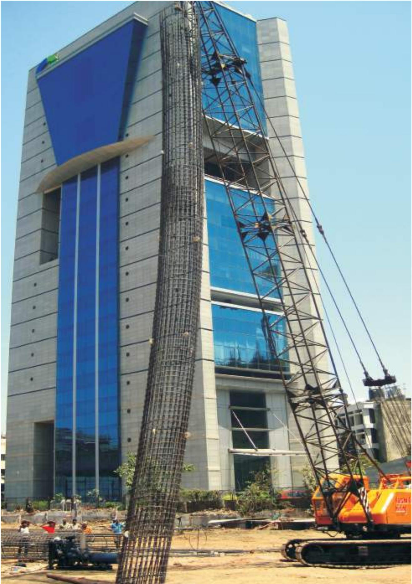
Cage Centring of 1500 mm Diameter of pile (22 to 28 mtr. Depth) at Worli Site, **OBEROI REALTY LTD**
