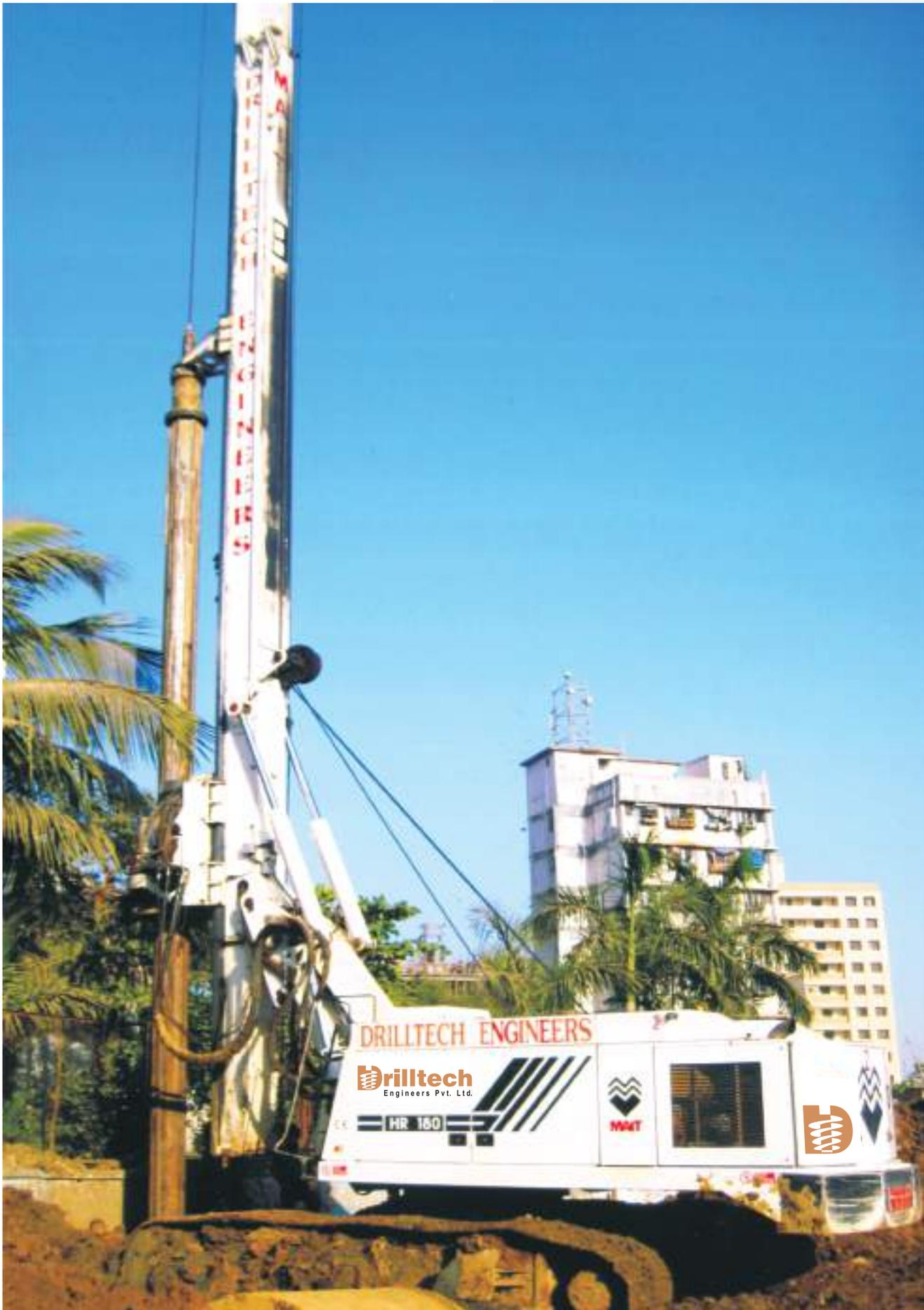
750 Numbers of piles, Depth 22-28 mtr. Having diameter (1200 mm - 1500 mm) by Hydraulic Rig HR-180.
