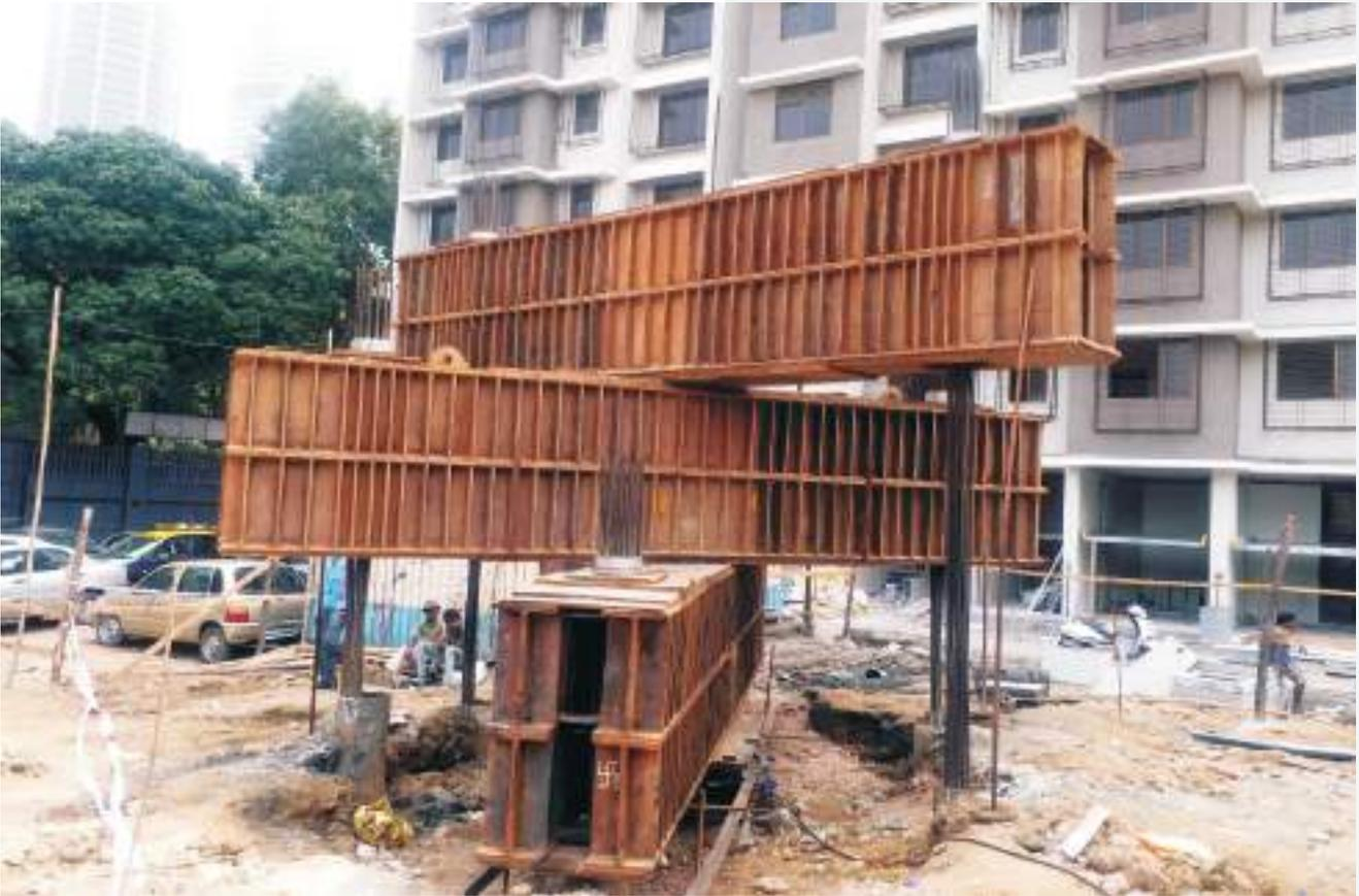
TATIC LOAD TEST of Foundation pile ( 600 mm & 700 mm diameter), Depth - 12 mtr., at Sunteck City, Phase I and Phase II, Naigaon, **SUNTECK REALTY LTD.**
