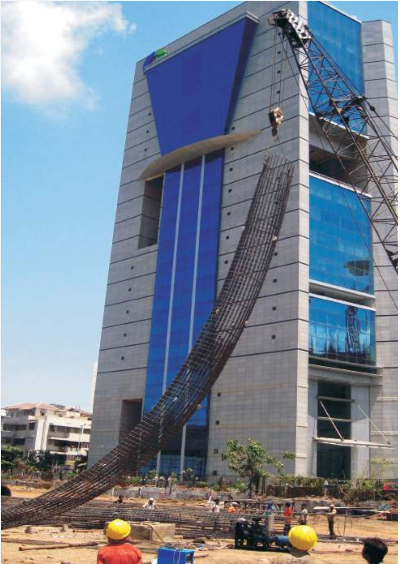
Cage Lifting of 1500 mm diameter of pile (25 mtr. Depth) at Worli Site, **OBEROI REALTY LTD.**
