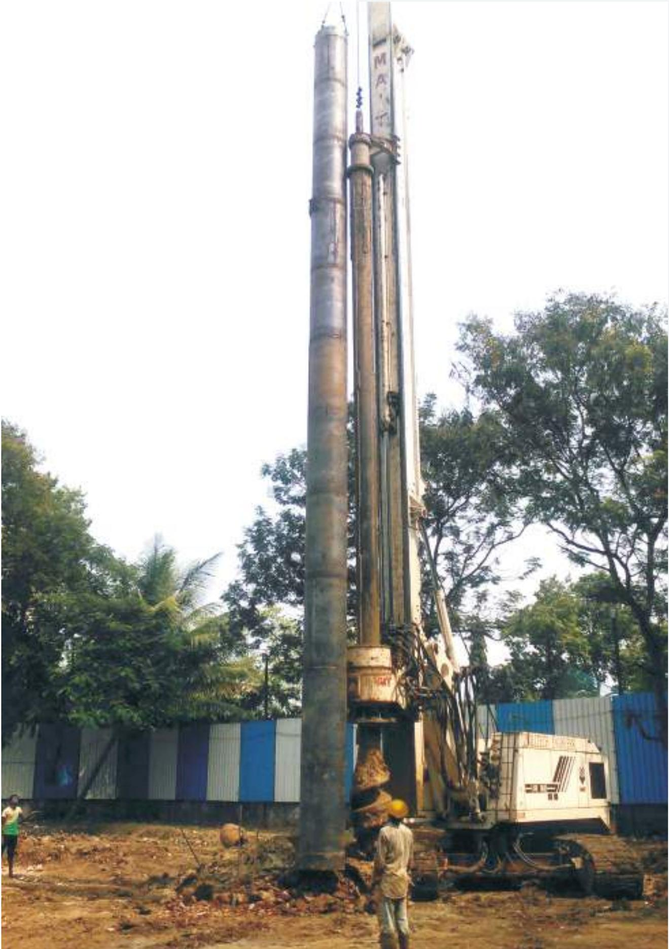
M.S.Liner Driven and Fixing for 700 mm Diameter of Pile at Yari Road, Versova, **PATEL REALTY**
