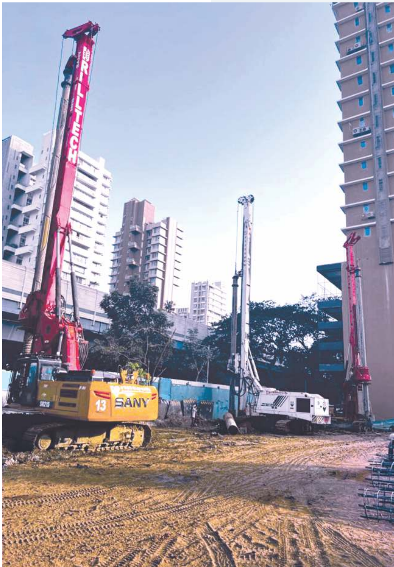
200 NOS. OF SHORE PILE, 600 MM DIAMETER, AT MATUNGA, GOSHAR ALLIANCE LLP.
