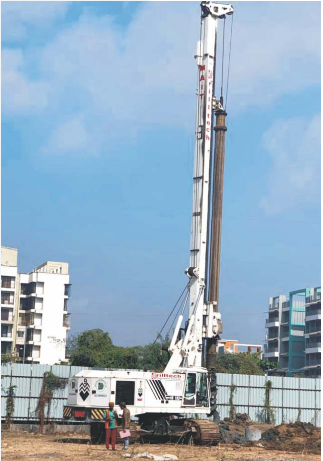
360 NOS. OF PILE, 700 MM DIAMETER. 18 MTR. DEPTH AT TURBHE - HINDUSTAN PLATINUM PVT. LTD.
