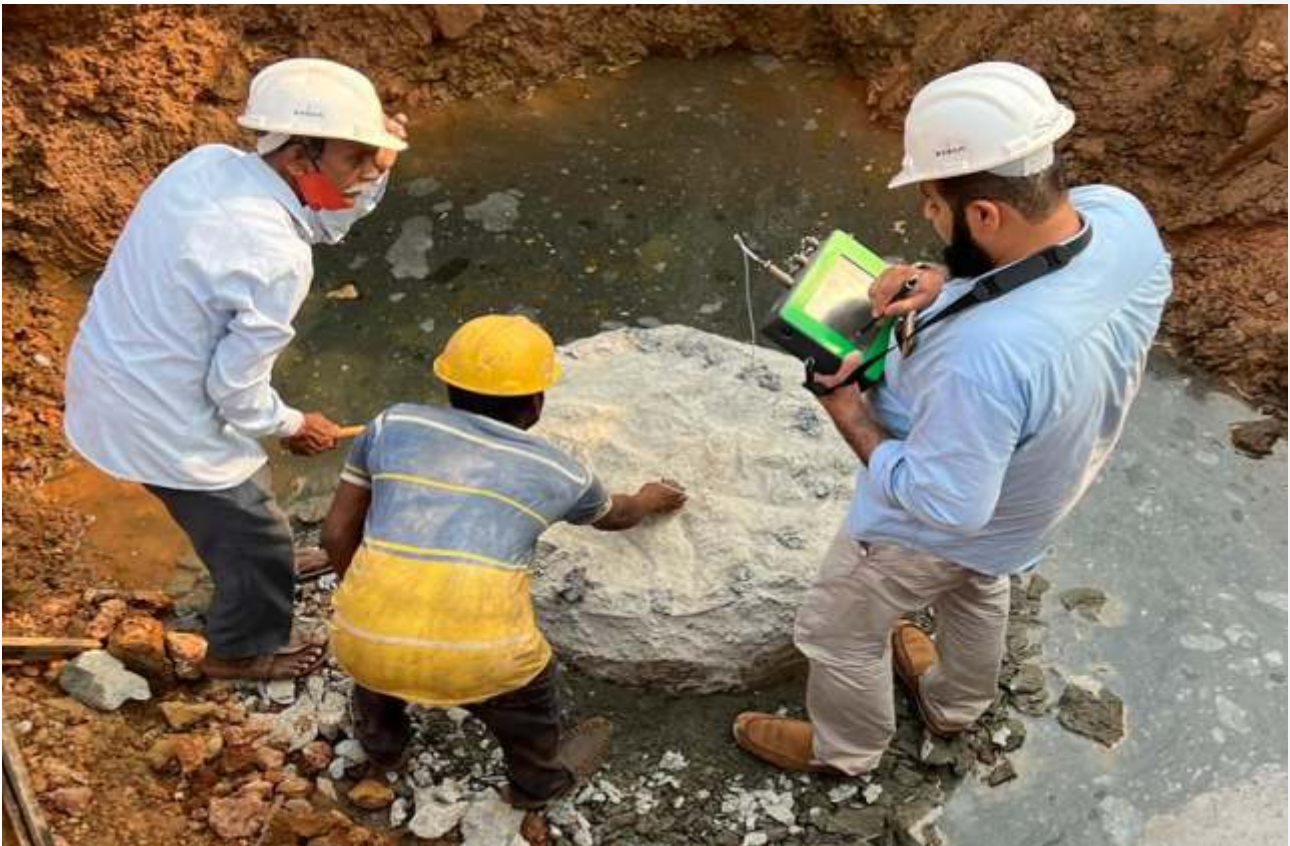
INTEGRITY TEST AT PANJIM GOA - DLF.
