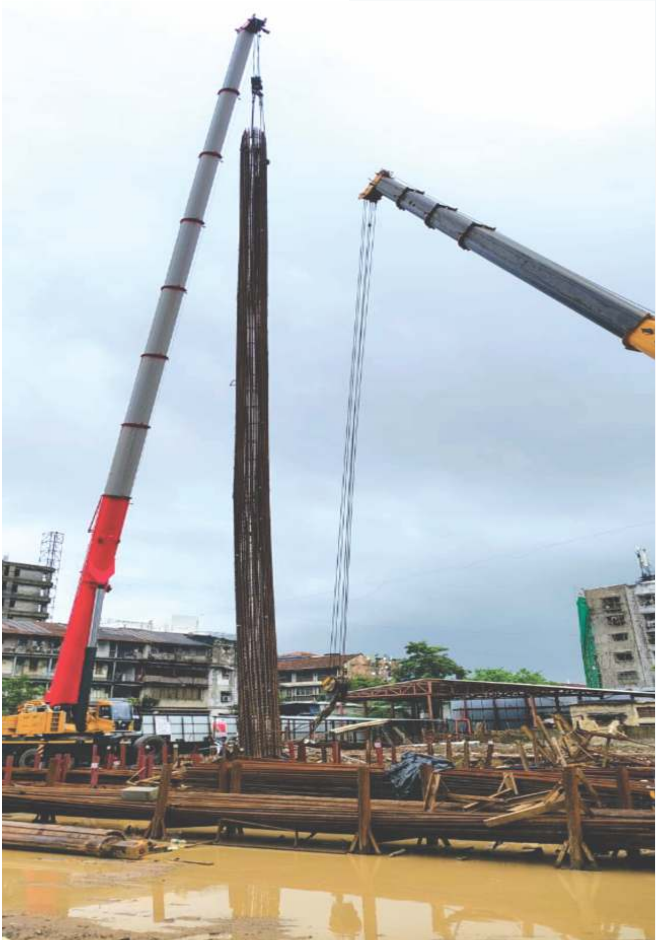
CAGE LIFTING OF 1200 MM DIAMETER OF PILE, 36 MTR. DEPTH, 25 M. TON AT CHARNI ROAD, MICL GROUP.
