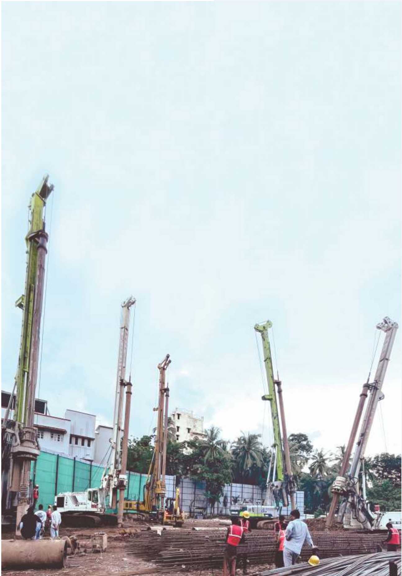
517 NOS. OF PILE, 600 & 700 MM DIAMETER, 16 MTR. DEPTH AT VILE PARLE MAN INFRA JADE PARK, MICL GROUP.
