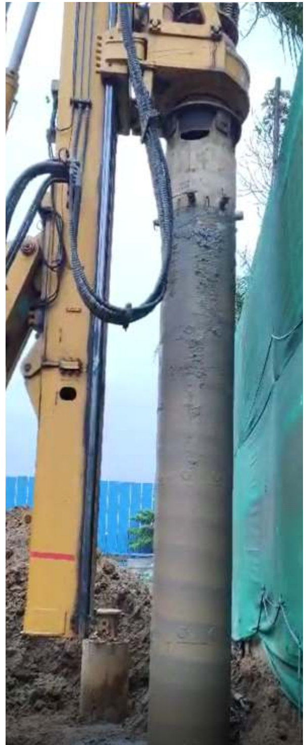
DOUBLE WALL CASING METHOD AT VERSOVA GALANI HOUSE, LANDMARK GROUP.
