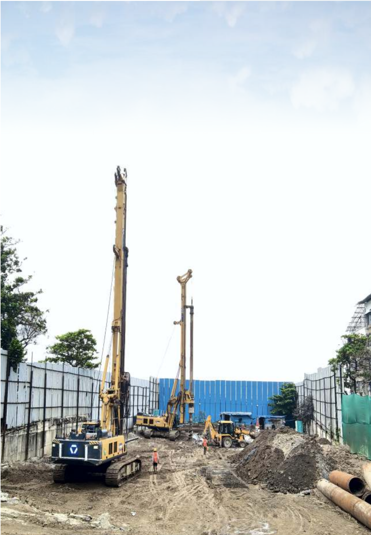
DOUBLE WALL CASING METHOD 280 NOS. OF PILE, 800 MM DIAMETER, 24 MTR. DEPTH AT VERSOVA GALANI HOUSE, LANDMARK GROUP.
