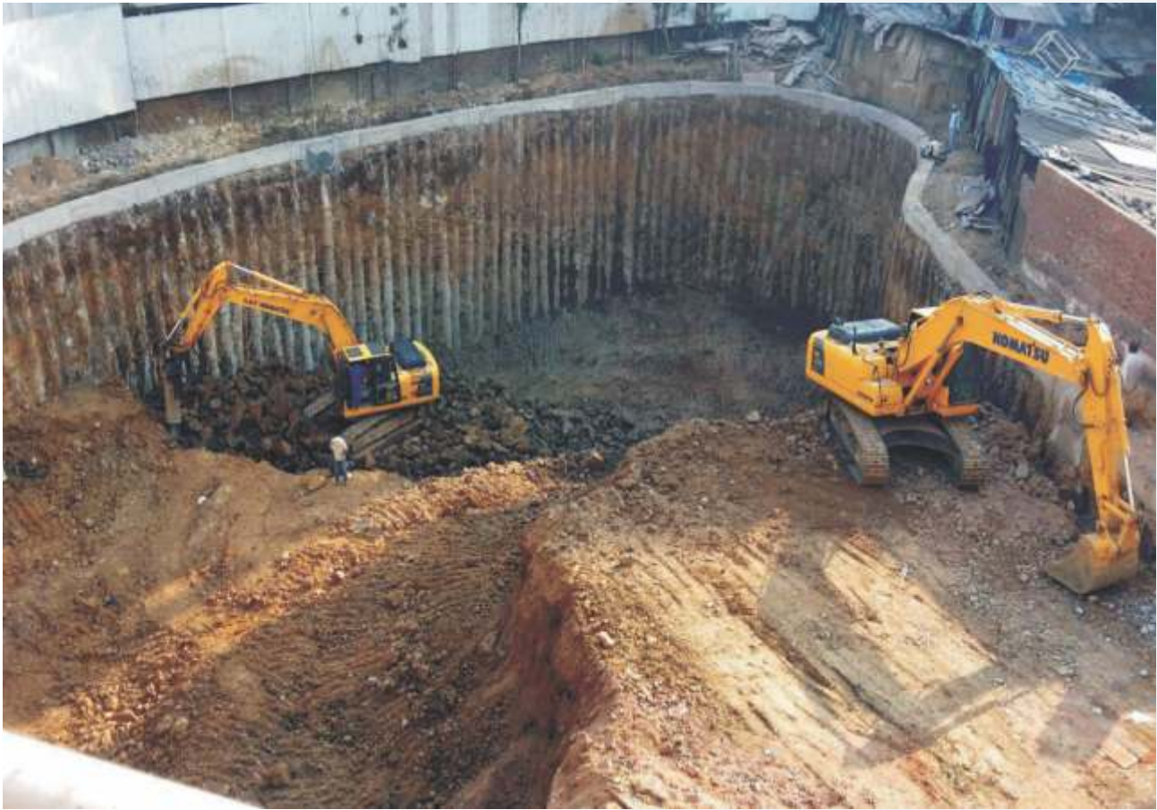
305 PILE OF BASEMENT WORK AFTER EXCAVATION OF PLOT AT CHAKALA SITE
