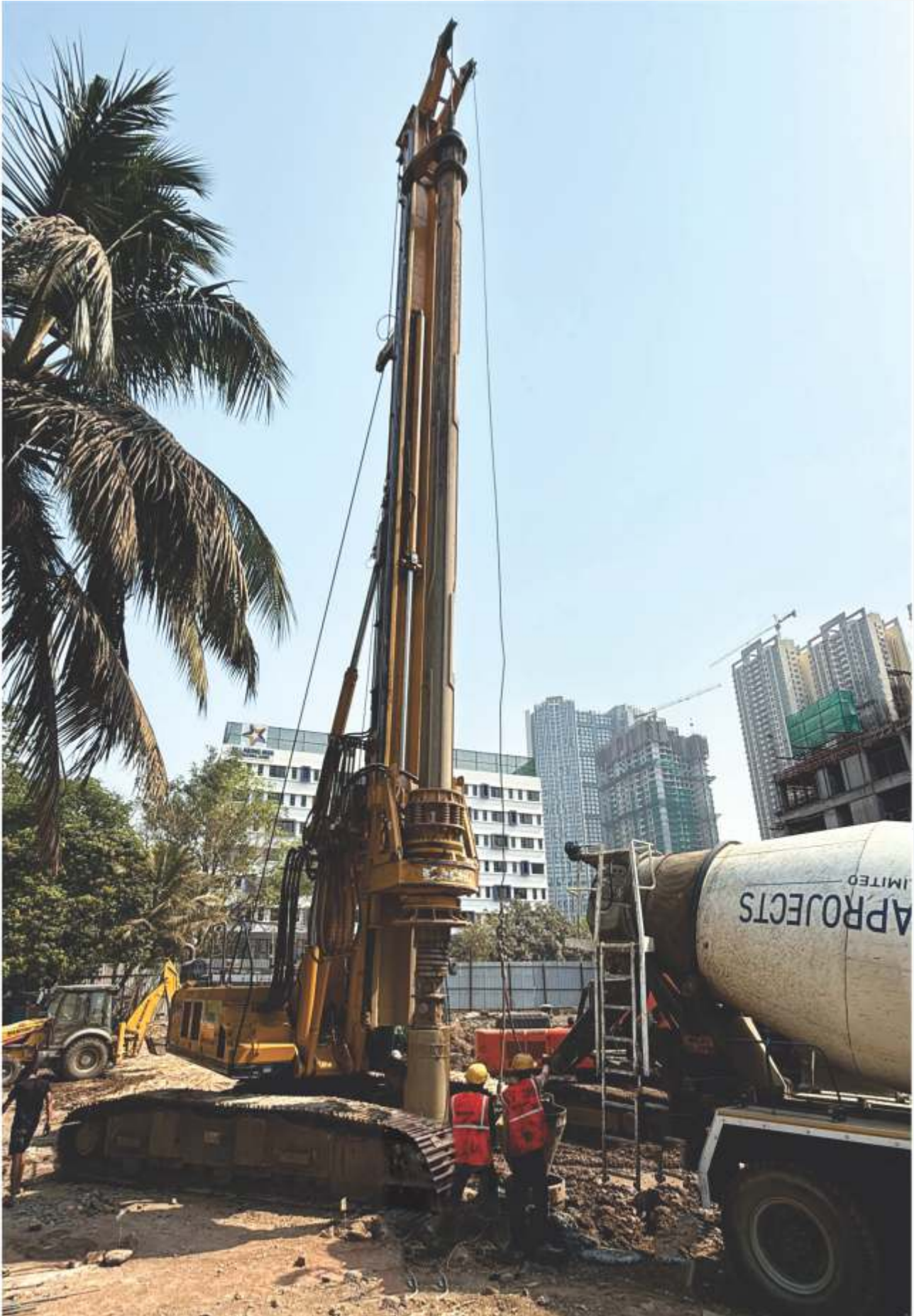
90 NOS. OF PILE, 600 MM DIAMETER, 10 MTR. DEPTH AT MULUND, ATUL INFRA.
