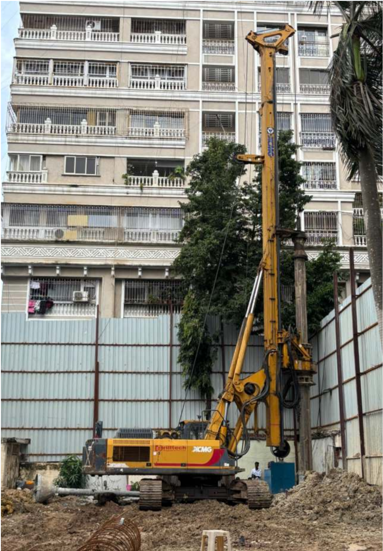
121 NOS. OF PILE, 600 MM DIAMETER, 9 MTR. DEPTH AT BANDRA - APILITE REALTY
