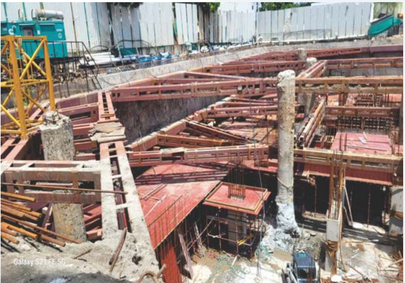
160 TON STRUT WORK AT OCEANA, SHIVAJI PARK DADAR, KOHINOOR PLANET CONSTRUCTION PVT. LTD.
