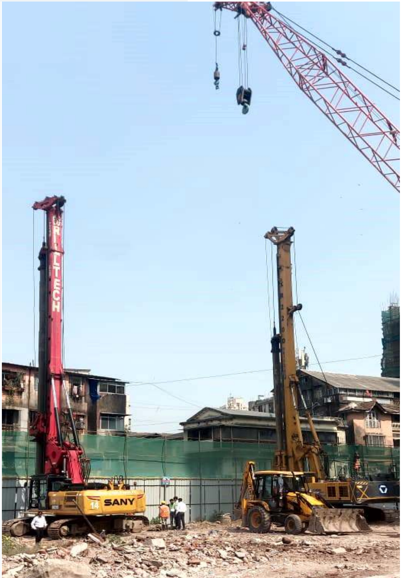
673 NOS. OF PILE, 600 & 800 MM DIAMETER, 16 MTR. DEPTH AT CHARANI ROAD SHAPOORJI PALLONJI REAL ESTATE, ODDYSSY PROJECT.
