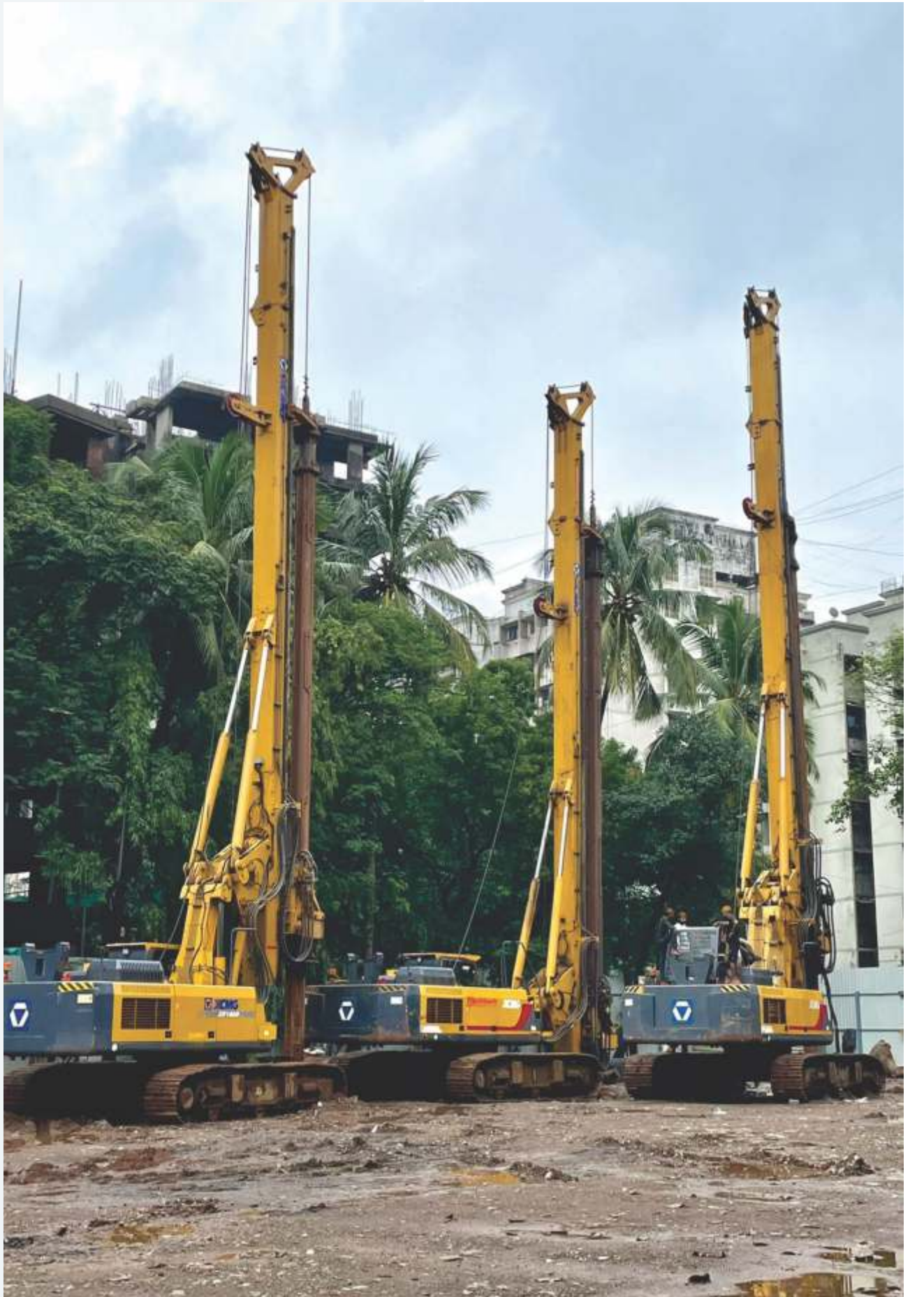
400 NOS. OF PILE, 15 MTR. TO 18 MTR. DEPTH AT GHATKOPAR, GOSHAIR ALLIANCE.
