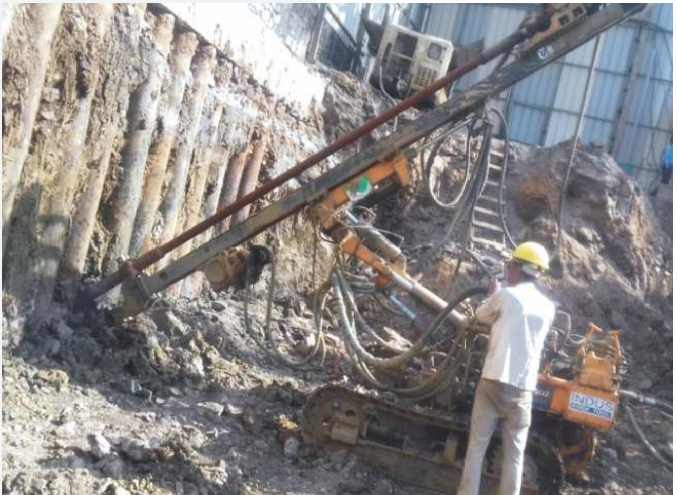
INCLINED ROCK ANCHORS AT SANJOG, KALPATARU.
