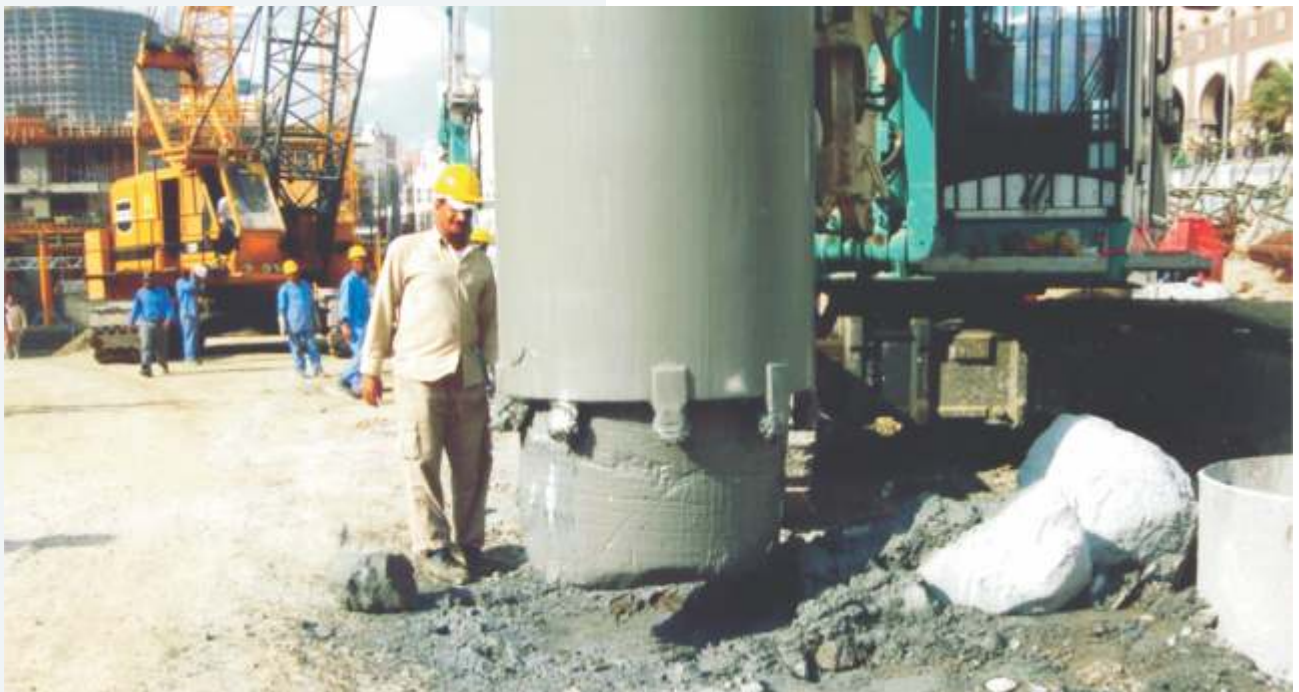
CORE CUTTING (BLACK BASALT)
