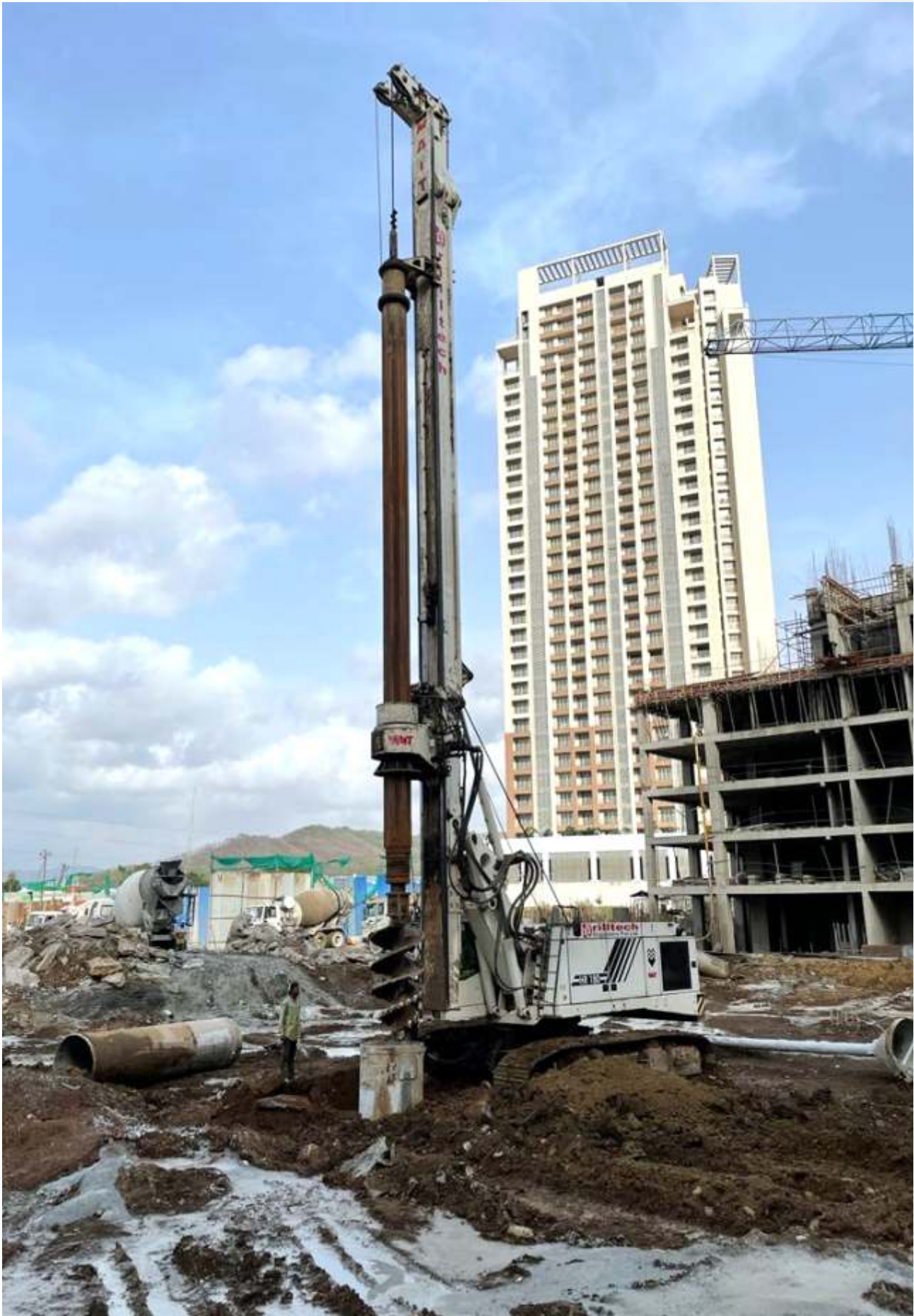
320 NOS. OF PILE, 1000 MM DIAMETER, 16 MTR DEPTH AT PANVEL - INDIA BULLS.
