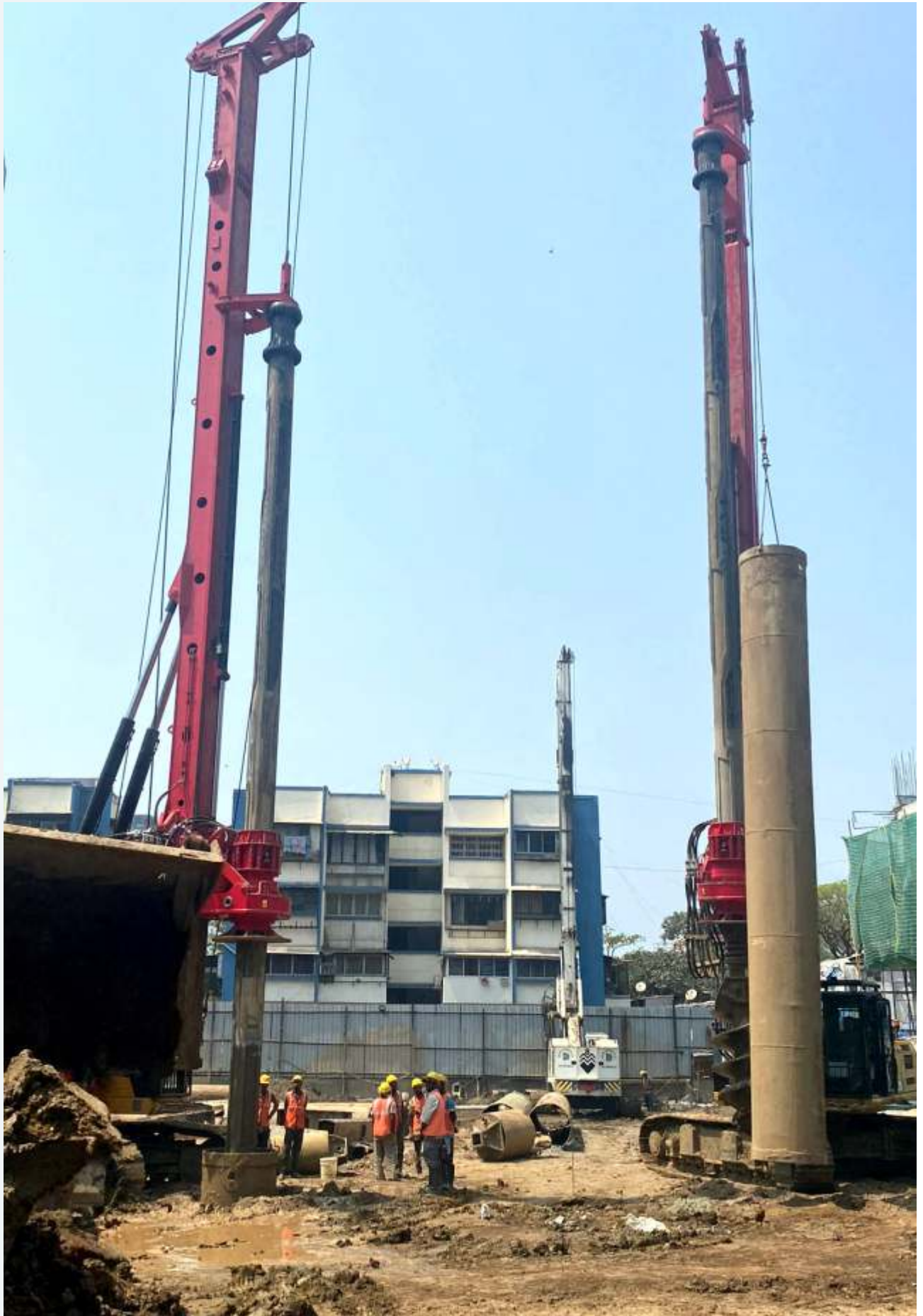
532 NOS. OF PILE, 800 & 1000 MM DIAMETER, 16 TO 18 MTR. DEPTH AT MAHIM, MIDTOWN BAY, PRESCON.
