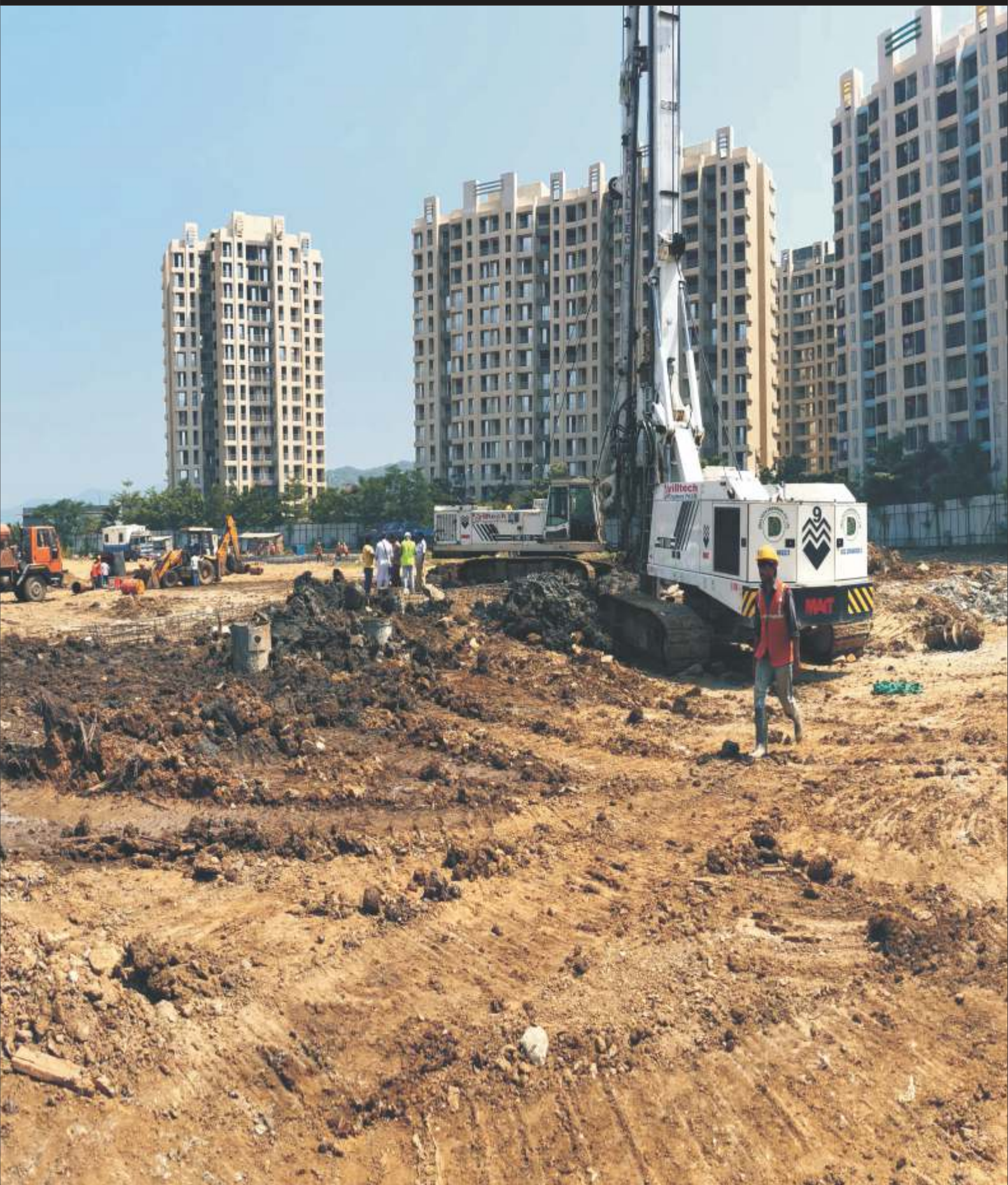
FOUNDATION PILE AT SUNTECK CITY, PHASE I AND PHASE II.
