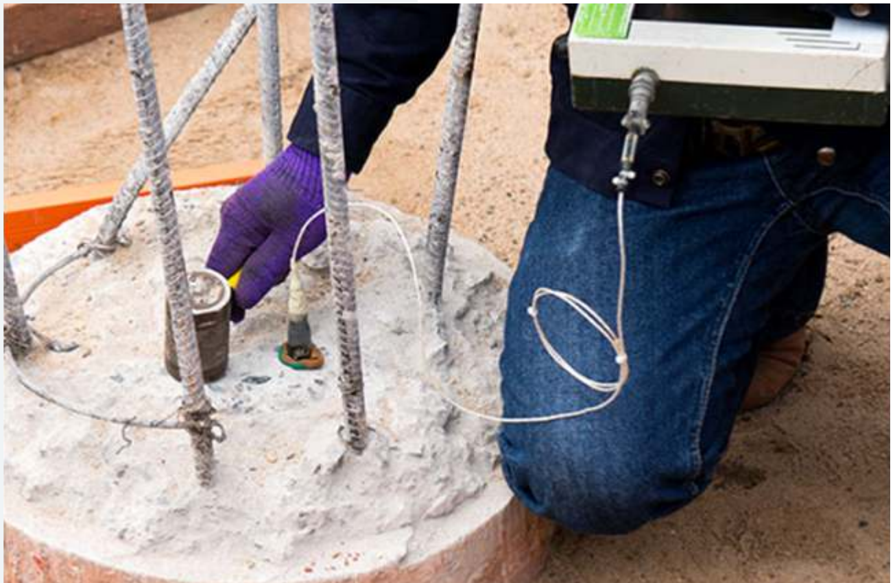
PILE INTIGRITY TEST FOR 3000 NOS. OF FOUNDATION PILE ( 600 MM & 700 MM DIAMETER), DEPTH - 12 MTR., AT SUNTECK CITY, PHASE I AND PHASE II, NAIGAON, SUNTECK REALTY LTD.
