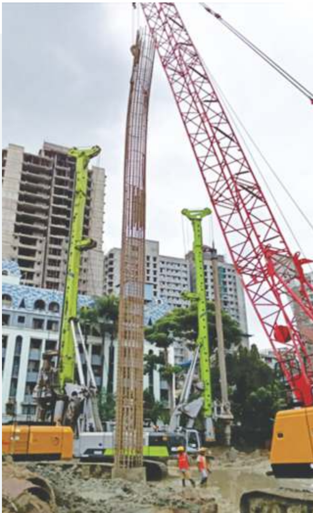
INSTALLATION OF STEEL CAGE AT CHARNI ROAD, MICL GROUP.
