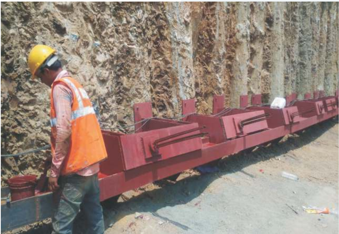
WALLER BEAM FABRICATION WITH STRESSING TEST COMPLETE AT BHANDUP WEST
