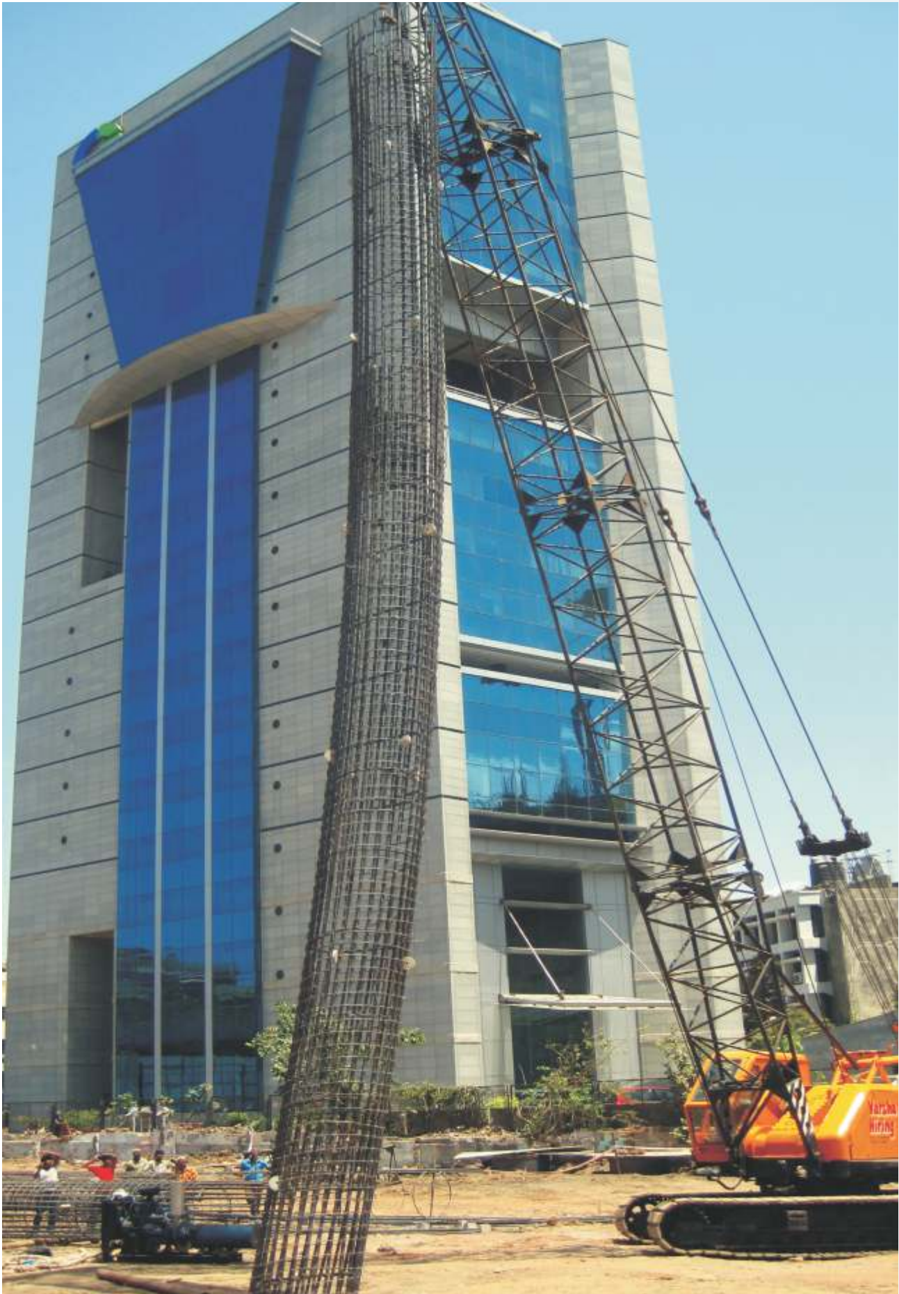
CAGE LIFTING OF 1500 MM DIAMETER OF PILE, 22 MTR. TO 28 MTR. DEPTH AT WORLI - OBEROI REALTY LTD.
