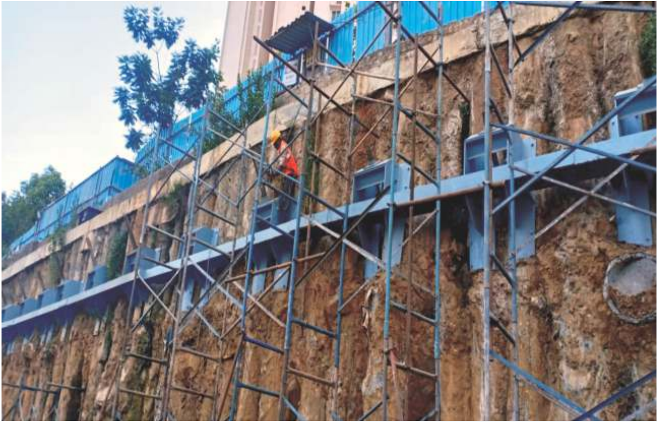
INCLINED ROCK ANCHORS AT THANE (WEST) , PURANIK BUILDERS LTD.
