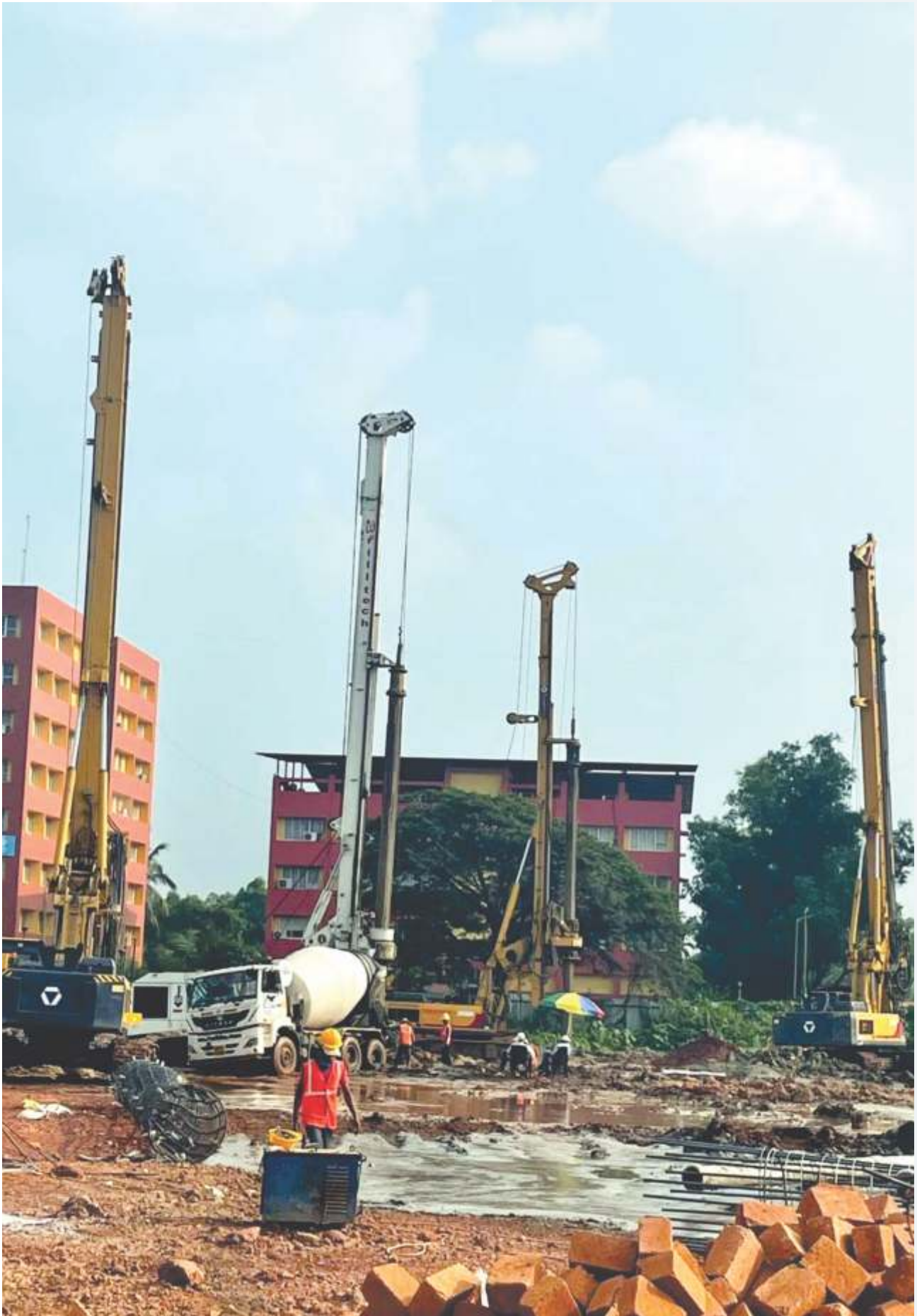
433 NOS. OF PILE, 1000 MM DIAMETER, 26 TO 32 MTR. DEPTH AT PANJIM GOA - DLF
