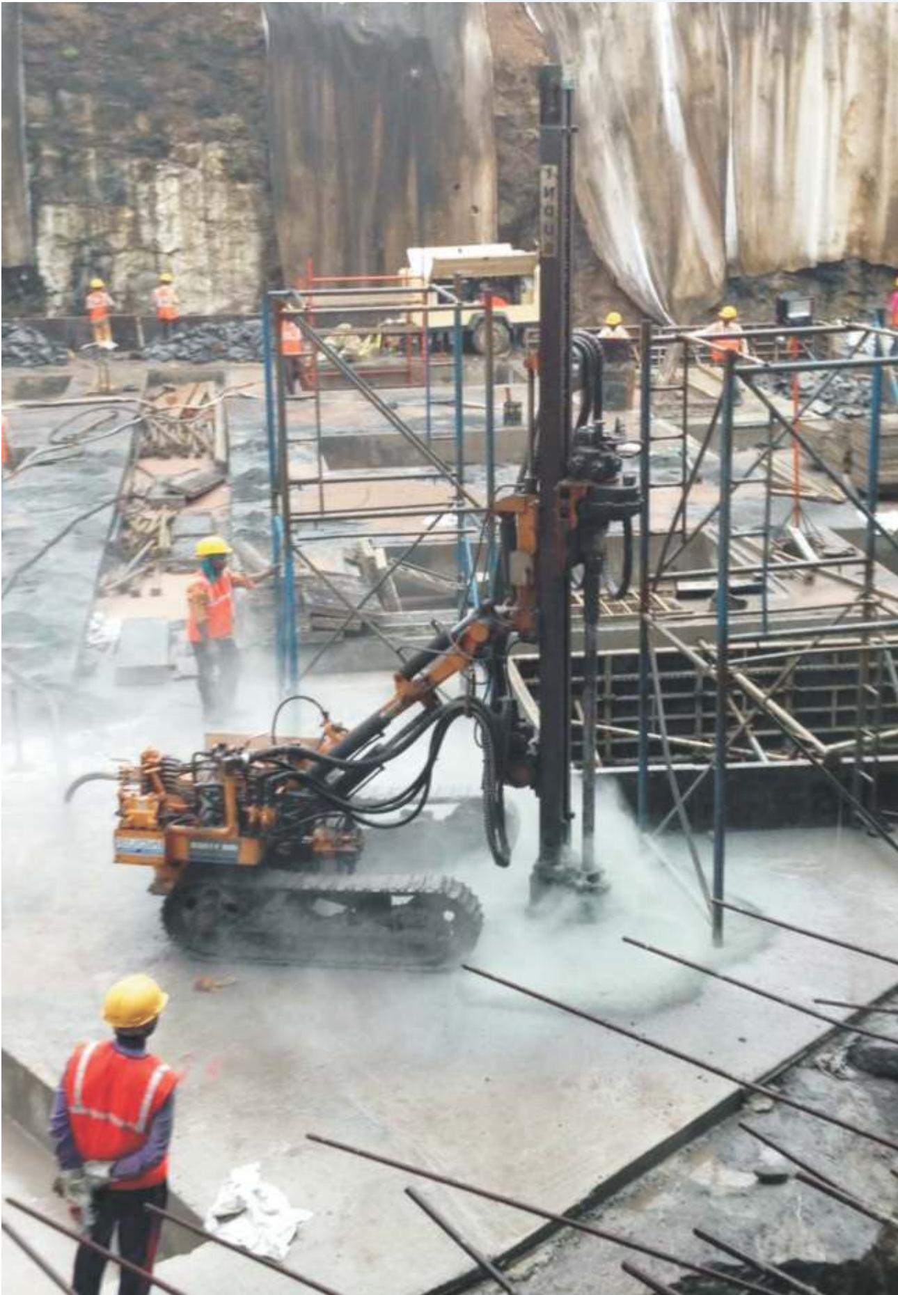
PASSIVE ROCK ANCHOR, 150 MM DIAMETER, AT MULUND SITE, OBEROI REALTY LTD.
