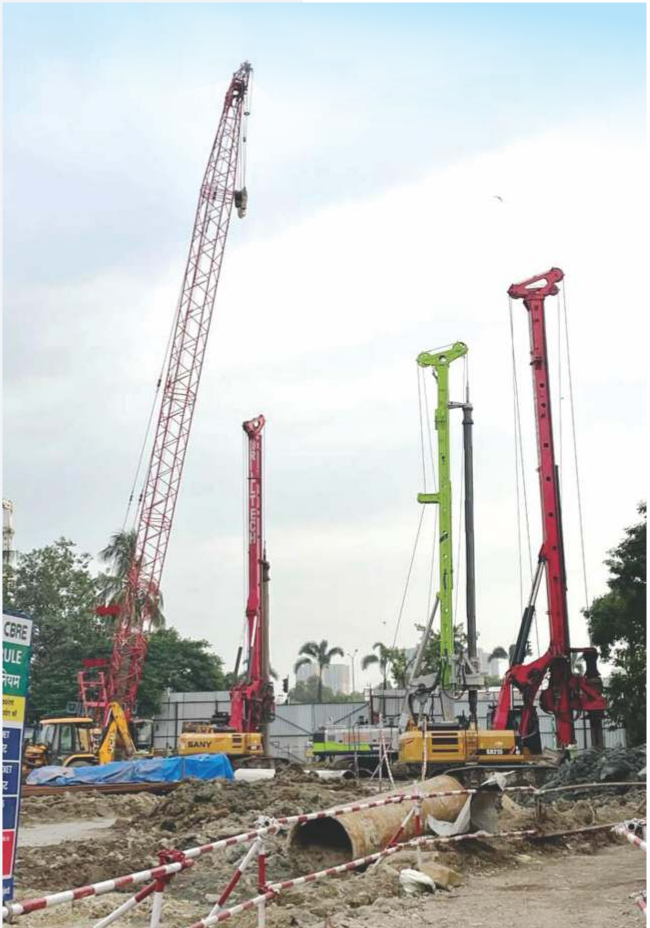
1200 NOS. OF PILE, 600 MM AND 800 MM DIAMETER, 25 MTR. DEPTH AT BKC, L&T CONSTRUCTIONS, PRESTIGE 101.
