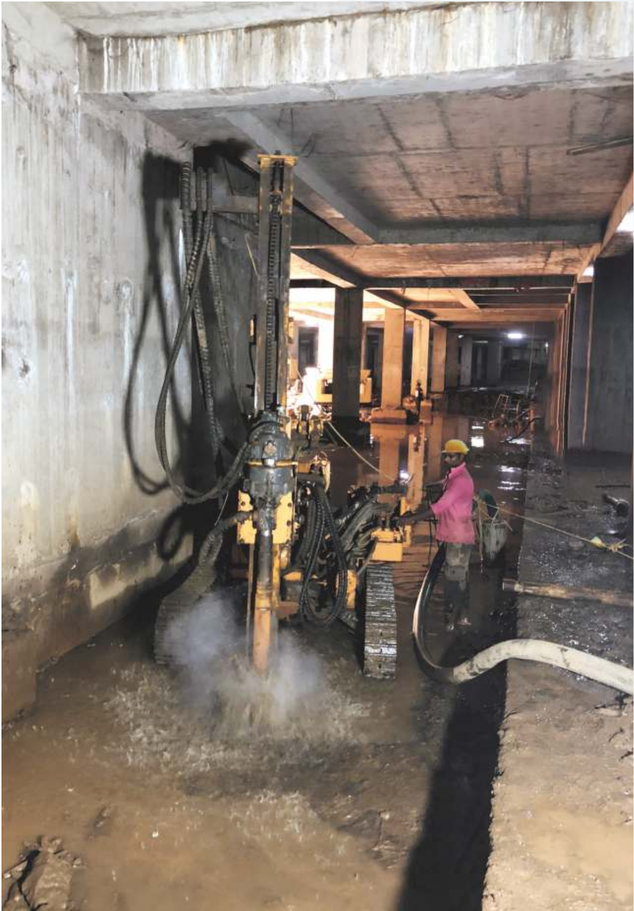
PASSIVE ROCK ANCHOR, 22 MM DIAMETER, AT GHATKOPAR (WEST), CHIRAG NAGAR, DAMJI SHAMJI SHAH GROUP.
