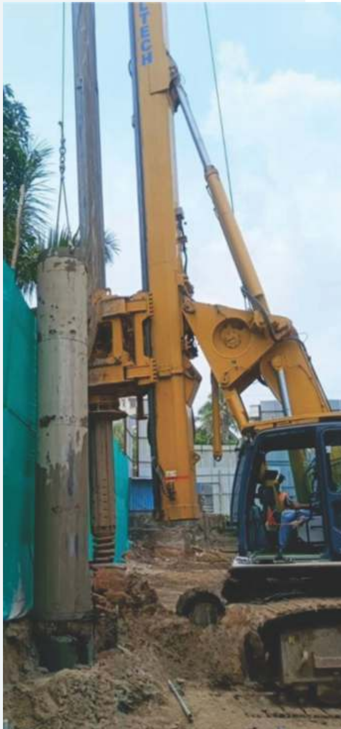
DOUBLE WALL CASING METHOD AT VERSOVA GALANI HOUSE, LANDMARK GROUP.
