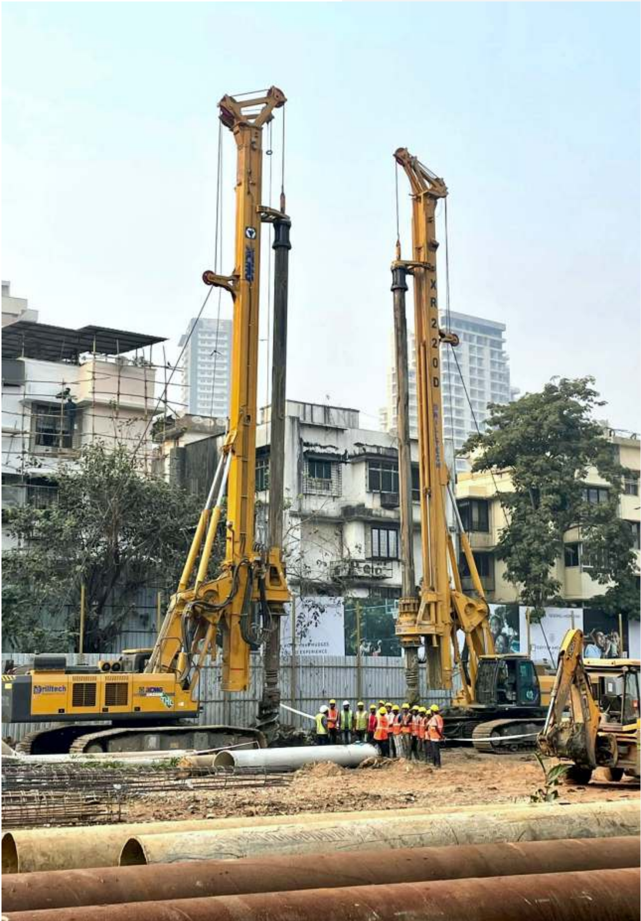
1455 NOS. OF SHORE PILE, 600 MM, 700 MM DIAMETER, 10 TO 13 MTR. DEPTH AT GODREJ HORIZON - WADALA.
