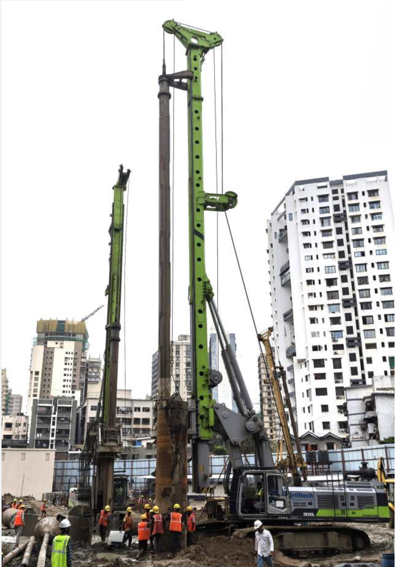
400 NOS. OF PILE, 1200 MM DIAMETER, 28 MTR. DEPTH AT CHARNI ROAD, MICL GROUP.
