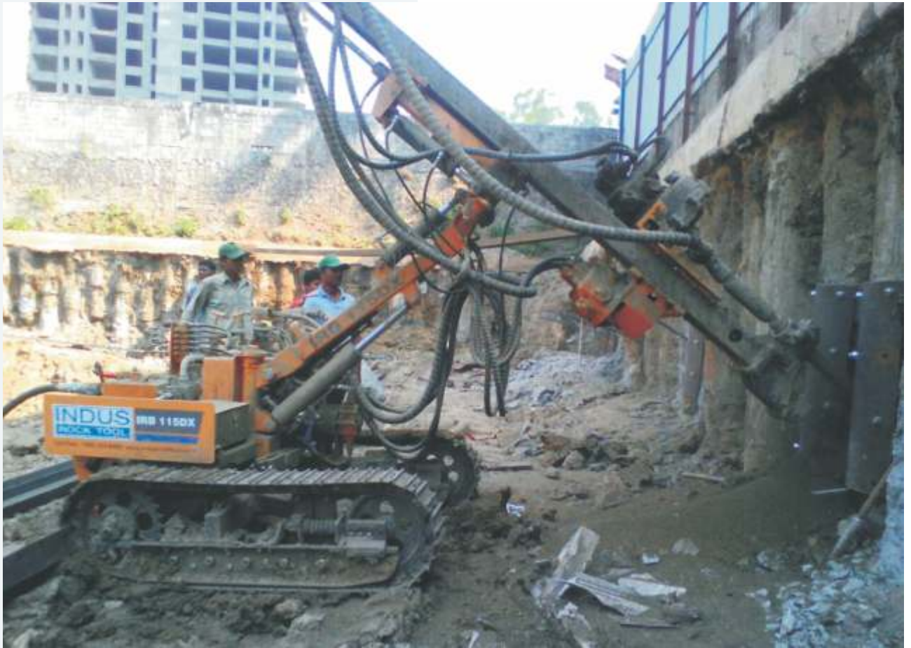
INCLINED ROCK ANCHORS AT BHANDUP, CEEAR LAND DEVELOPER
