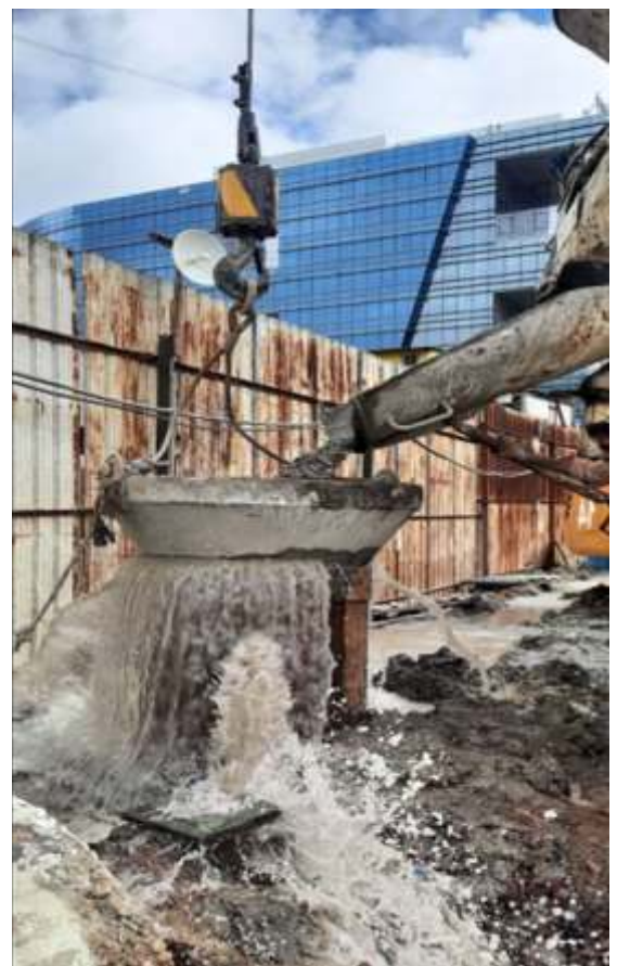
PILE CONCRETING
