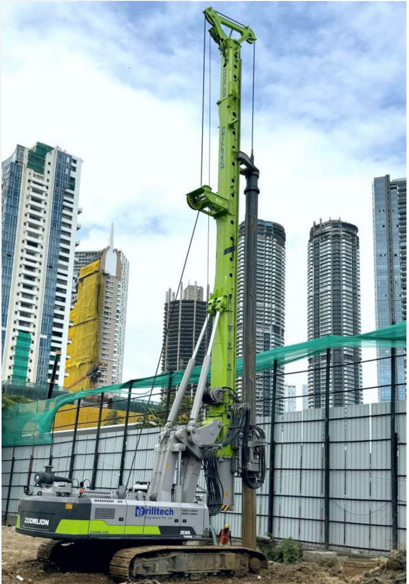
300 NOS. OF PILE, 800 & 1200 MM DIAMETER, 21 MTR. DEPTH AT WORLI - PRESTIGE NAUTILUS, PRESTIGE GROUP.
