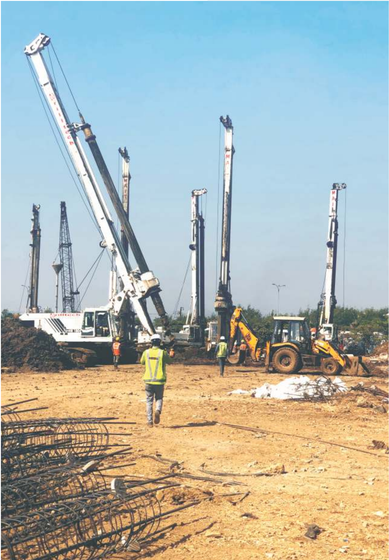
600 MM & 700 MM DIAMETER, 12 MTR. DEPTH, AT SUNTECK CITY, NAIGAON, SUNTECK REALTY LTD.
