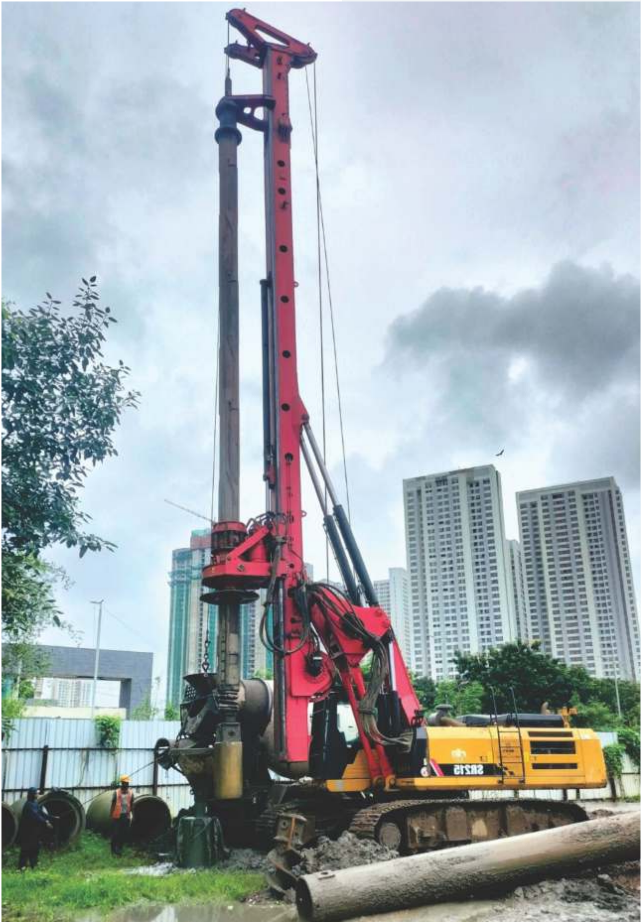
250 NOS. OF FOUNDATION PILE, 1000 MM & 800 MM DIAMETER, 17 MTR. DEPTH AT THANE, DOSTI REALTY.
