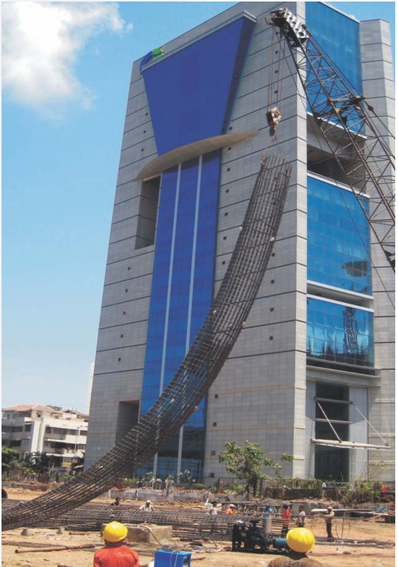
CAGE LIFTING OF 1500 MM DIAMETER, 800 NOS. OF PILE, 22 MTR. TO 28 MTR. DEPTH AT WORLI - OBEROI REALTY LTD.
