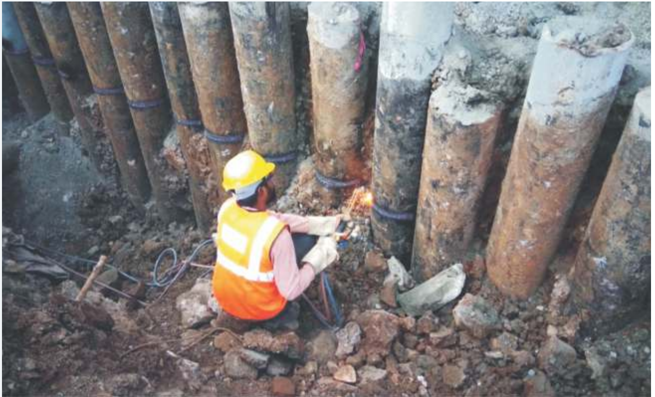
300 MM DIAMETER MICRO PILE LINER CUTTING
