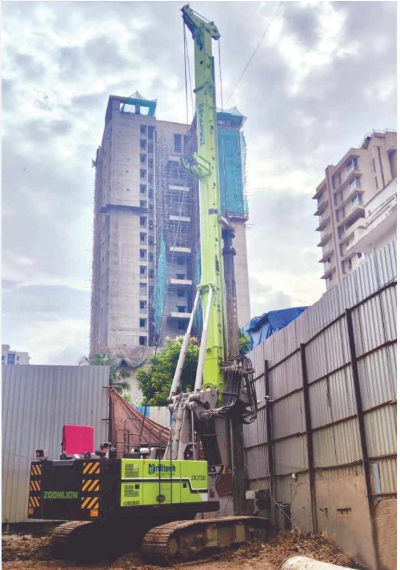
300 NOS. OF PILE, 600 MM DIAMETER, 11 MTR. DEPTH AT MATUNGAAMARAA, PRINCE CARE REALTY.
