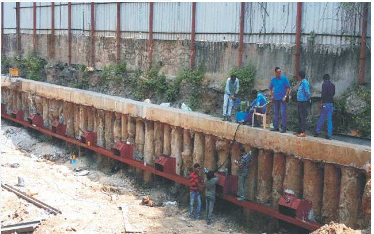
WALLER BEAM FABRICATION WITH STRESSING TEST COMPLETE AT BHANDUP (WEST).
