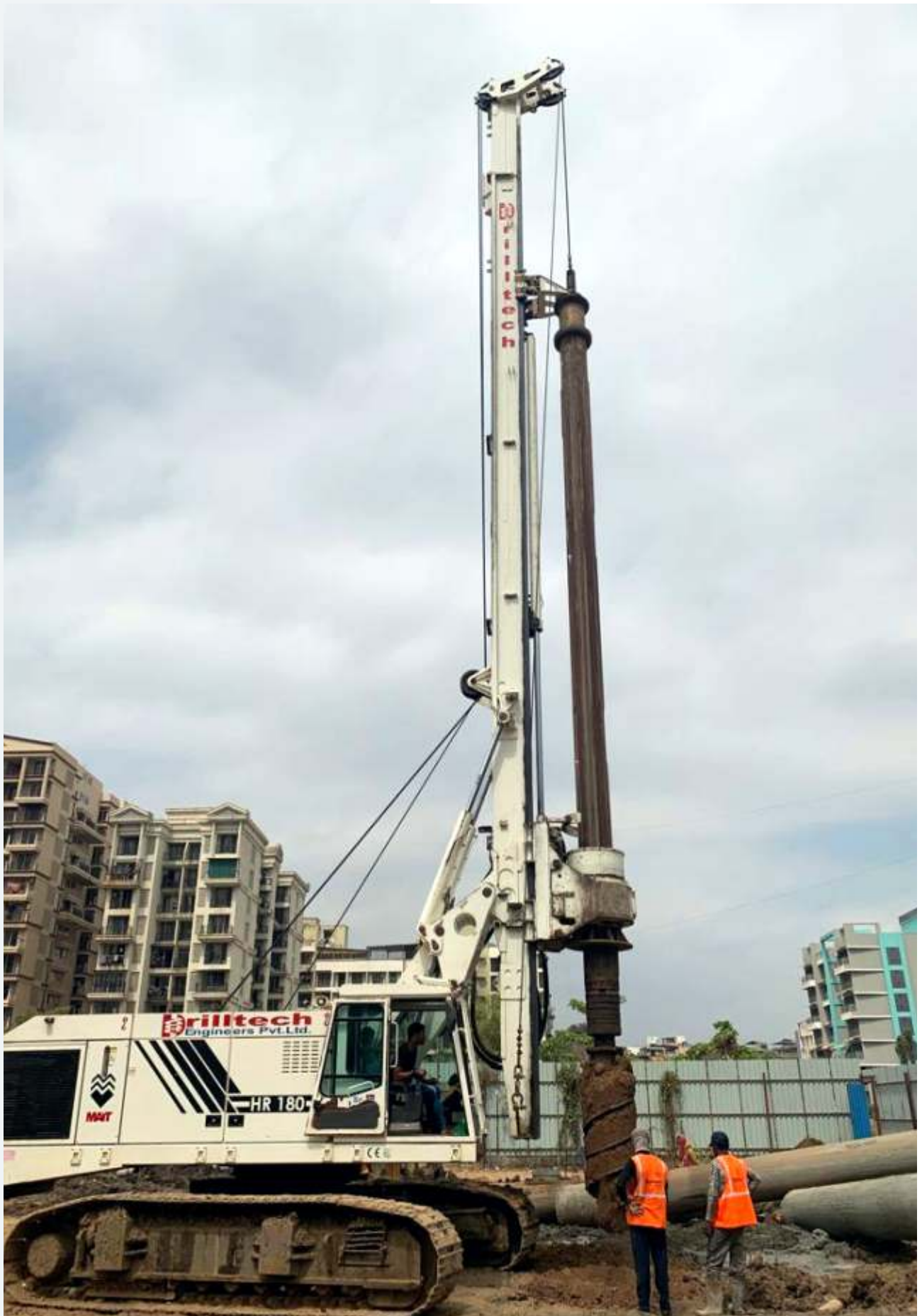
220 NOS. OF PILE, 600 MM, 700 MM AND 1000 MM DIAMETER. 22 MTR. DEPTH AT WADALA - CHANDAK GROUP.
