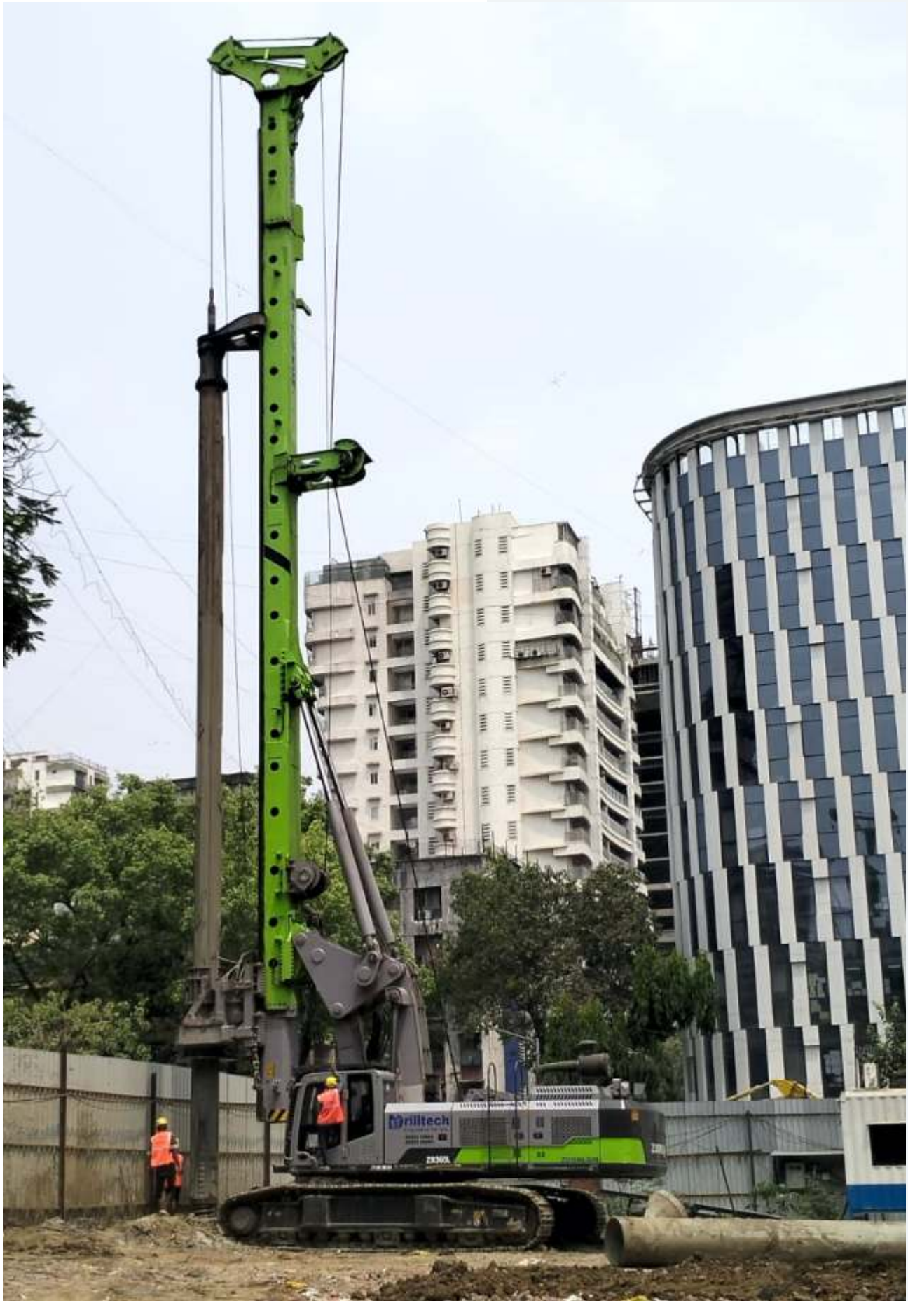
350 NOS. OF PILE, 700 MM DIAMETER, 24 MTR. DEPTH AT BANDRA - AJMERA LUKS REALTY.
