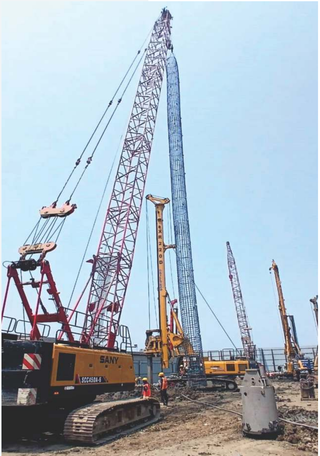
200 NOS. OF PILE, 1200 MM DIAMETER, 42 TO 45 MTR. DEPTH AT BHAYANDER NORTH WEST END, JP INFRA
