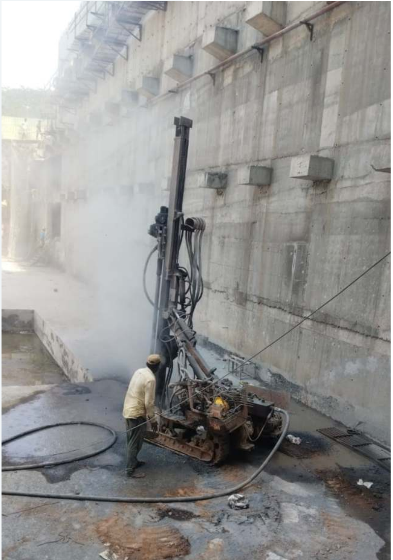
3000 NOS. PASSIVE ROCK ANCHOR, 200 MM DIAMETER, AT MIRA ROAD SITE, JP MALL, JP INFRA.
