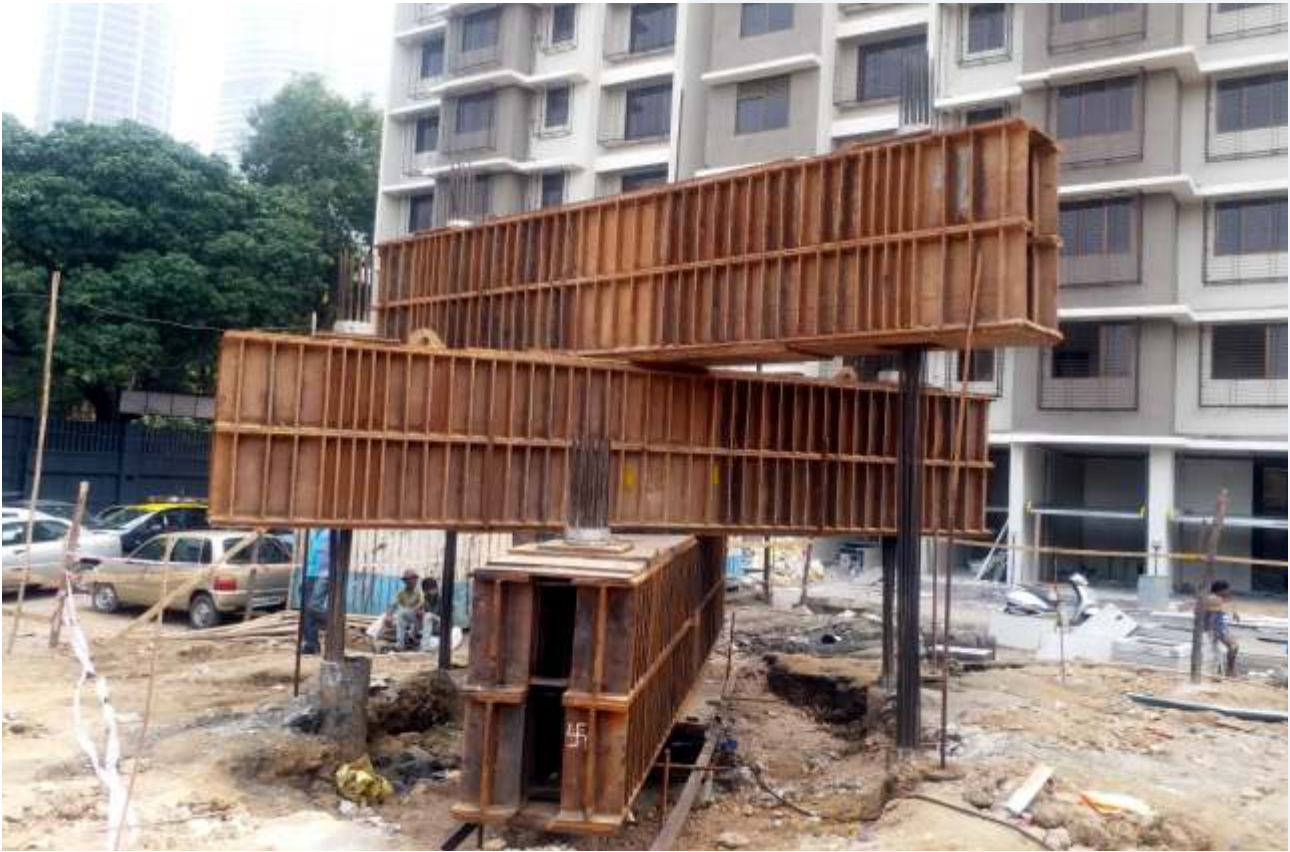
STATIC LOAD TEST OF FOUNDATION PILE, 600 MM & 700 MM DIAMETER, DEPTH - 12 MTR. AT SUNTECK CITY, PHASE I AND PHASE II, NAIGAON, SUNTECK REALTY LTD.
