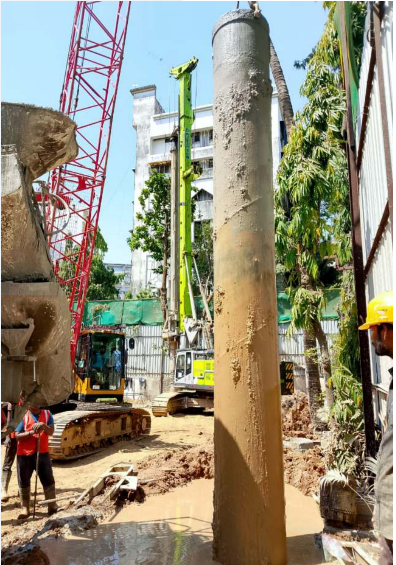
215 NOS. OF PILE, 600 MM DIAMETER, 27 MTR. DEPTH AT VILE PARLE NOTAN EDGE, NOTAN EMPRESS PVT LTD.
