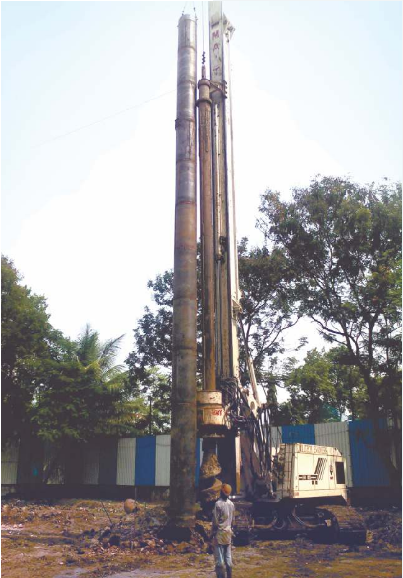
440 NOS. OF PILE, 700 MM DIAMETER, 18 MTR. DEPTH, 8 MM THICKNESS, PERMANENT MS CASING, AT YARI ROAD, VERSOVA, PATEL REALTY.
