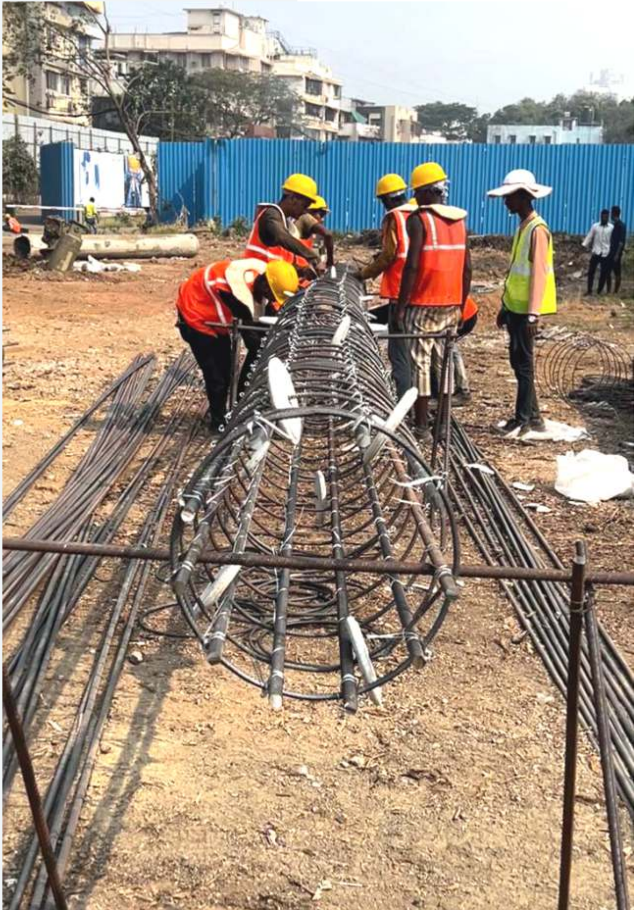
CAGE MAKING, 1455 NOS. OF SHORE PILE, 600 MM, 700 MM DIAMETER, 10 TO 13 MTR, DEPTH AT GODREJ HORIZON - WADALA
